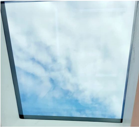
PROJECT PHOTOGRAPH A flat rooflight seen from the room below.
