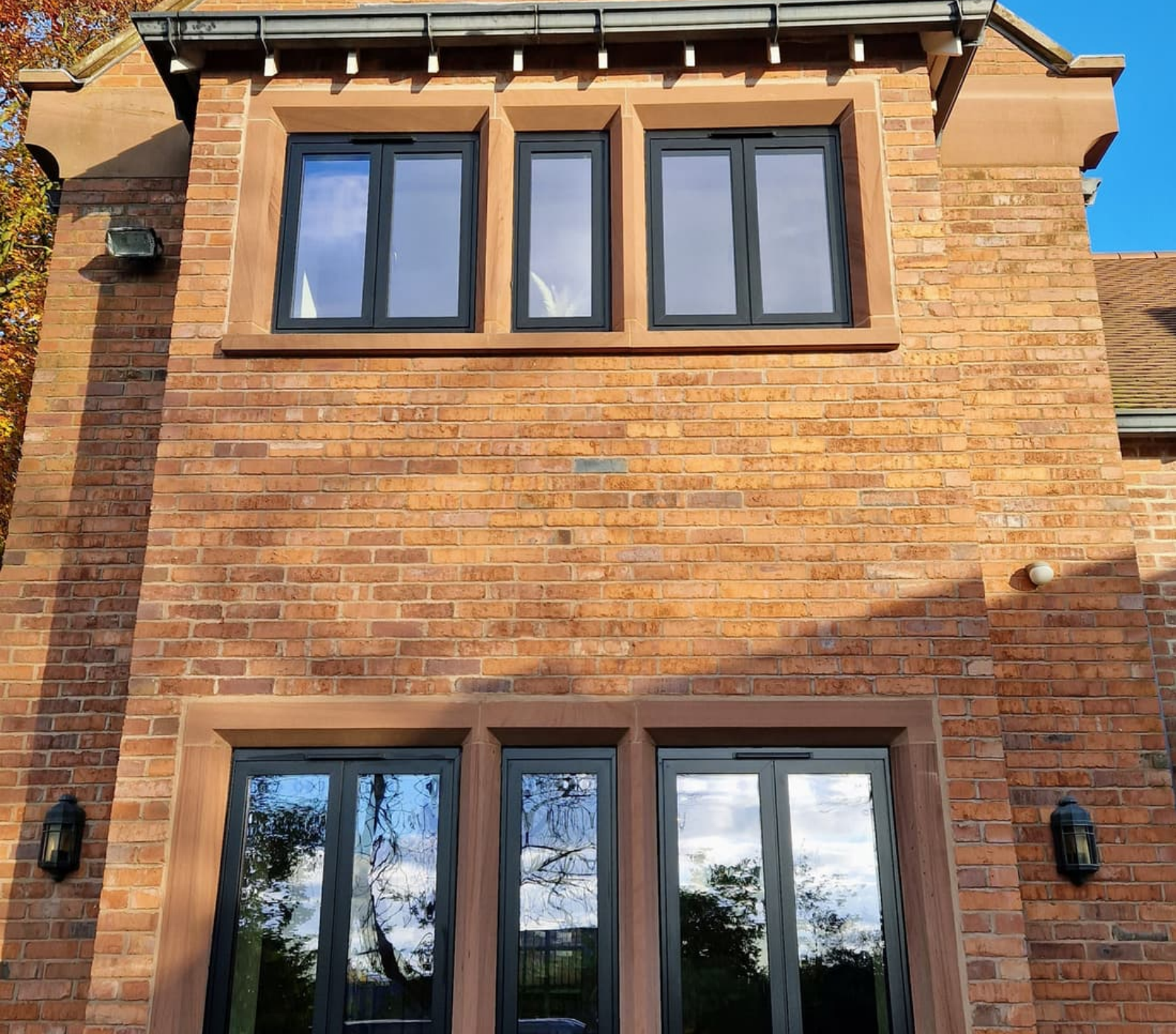
PROJECT PHOTOGRAPH Anthracite casement runs on both floors of a red brick gable, set into sandstone surrounds.
