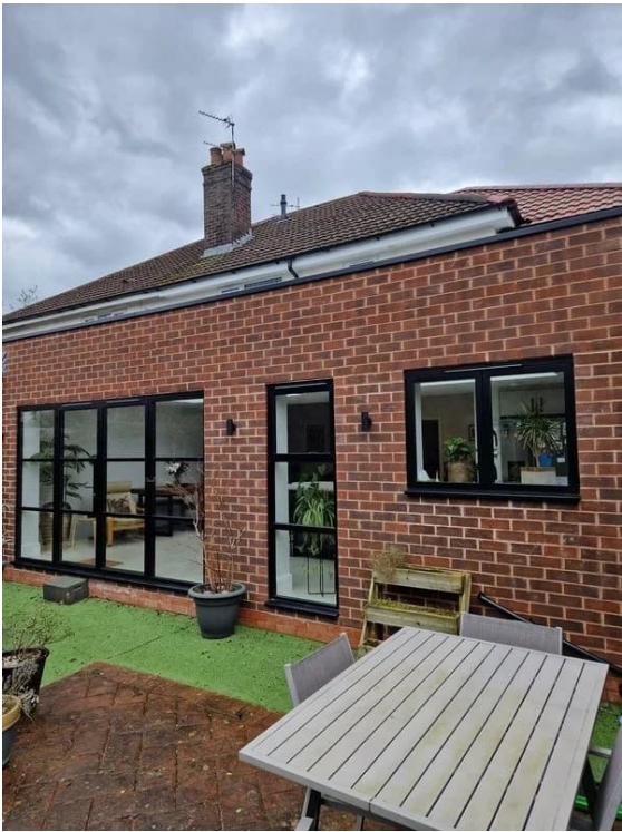
PROJECT PHOTOGRAPH A steel-look glazed screen, a glazed door and a window across one brick elevation.
