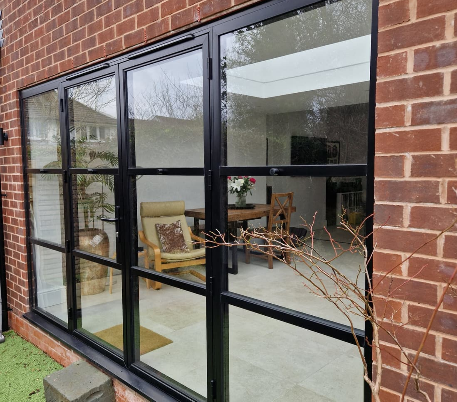
PROJECT PHOTOGRAPH A black heritage door set with glazing bars in a red brick elevation, with the dining room and a flat roof lantern showing through.
