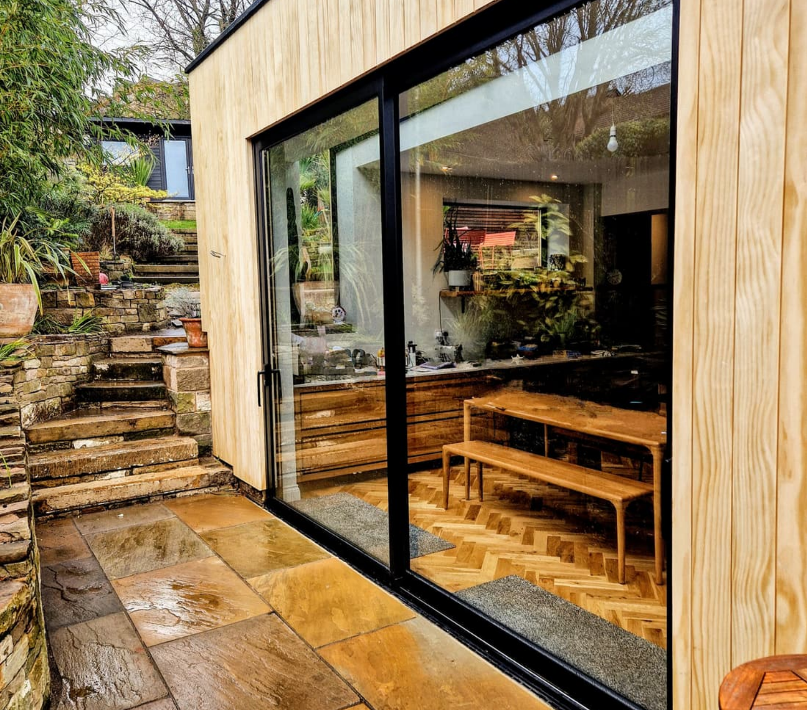
PROJECT PHOTOGRAPH A black sliding door in a timber clad extension, with wet sandstone flags outside and a herringbone floor within.
