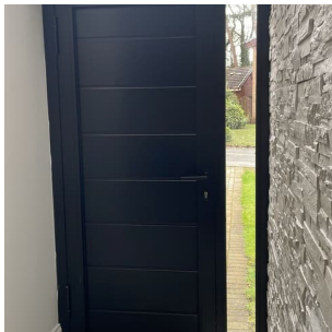
Entrance doors p . 14
