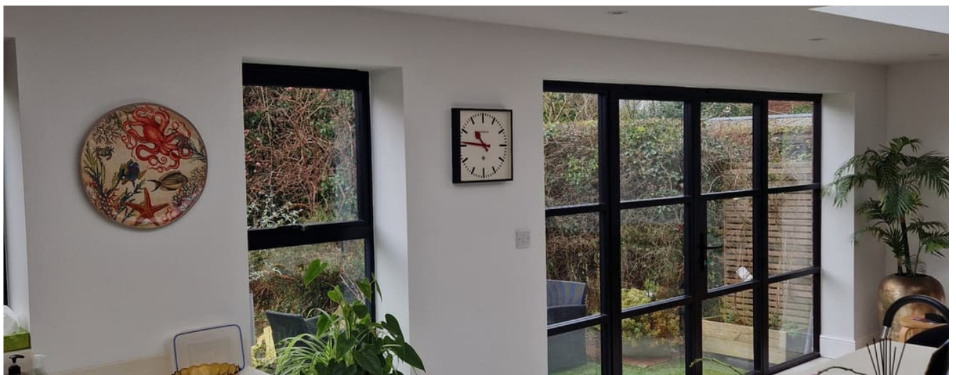
PROJECT PHOTOGRAPH A heritage screen and a tall narrow window with matching glazing bars, seen from inside.
