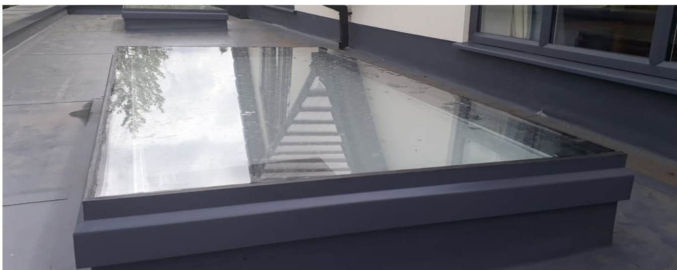
PROJECT PHOTOGRAPH An anthracite flat rooflight on a single-ply flat roof, seen across its kerb, with a second rooflight beyond.
