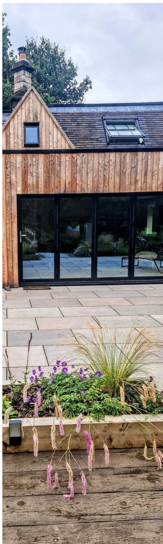
PROJECT PHOTOGRAPH Timber-clad extension, black aluminium bifolds, sandstone terrace.
