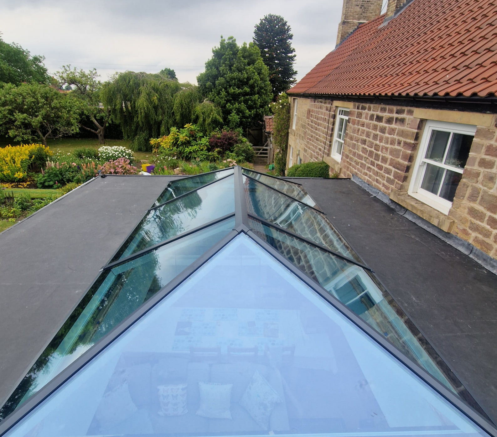
PROJECT PHOTOGRAPH A pyramid roof lantern on the flat roof of a stone cottage extension, with the garden and pantile roof behind.
