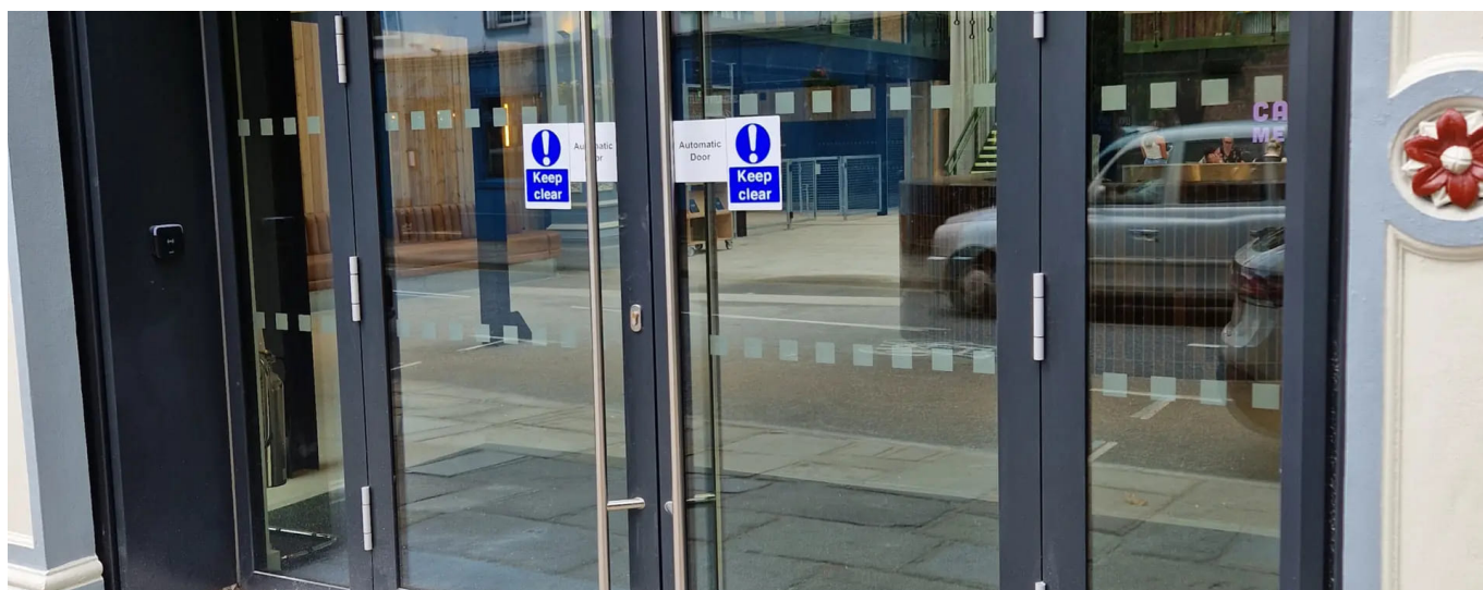
PROJECT PHOTOGRAPH The completed double entrance makes door handing, side-screen splits, threshold and hardware visible in one frame.
