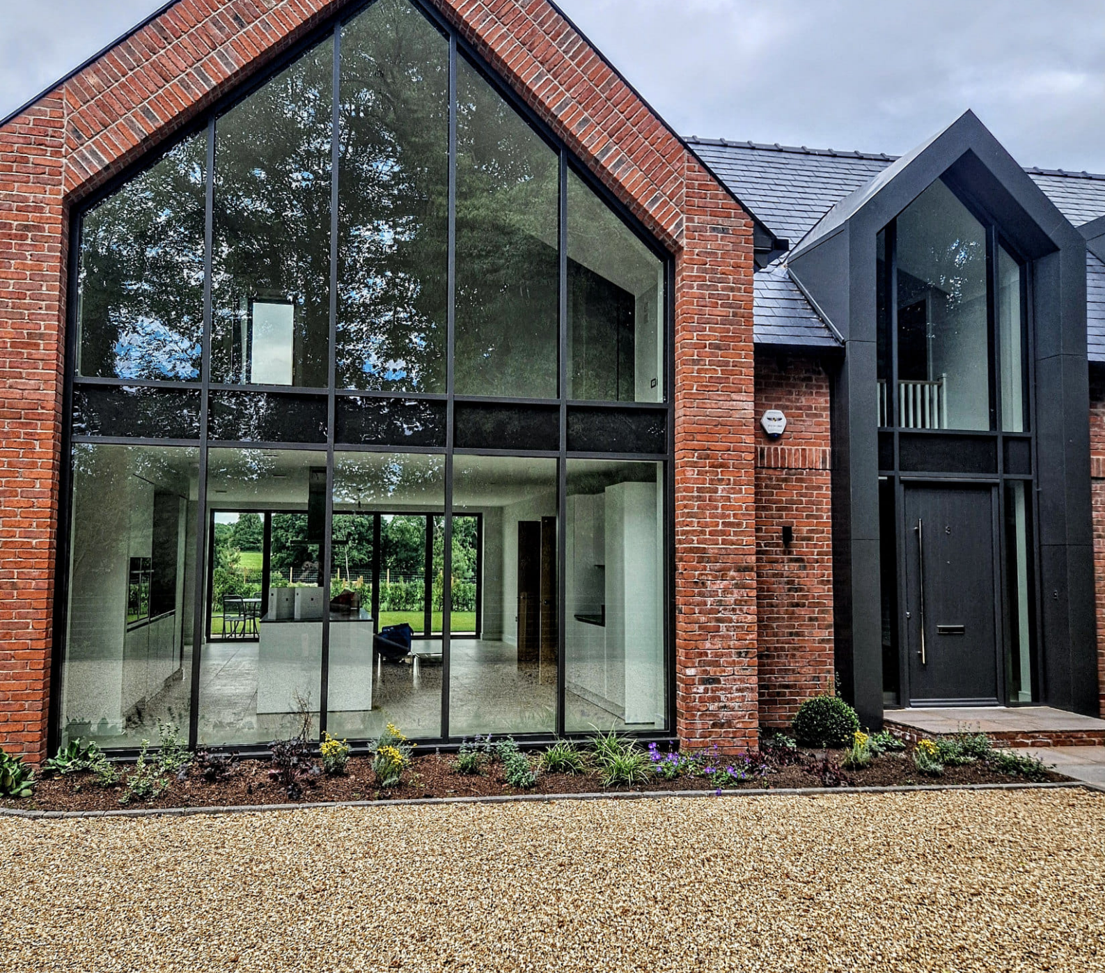
PROJECT PHOTOGRAPH A double height glazed gable in black aluminium, set into red brickwork with a slate roof alongside.
