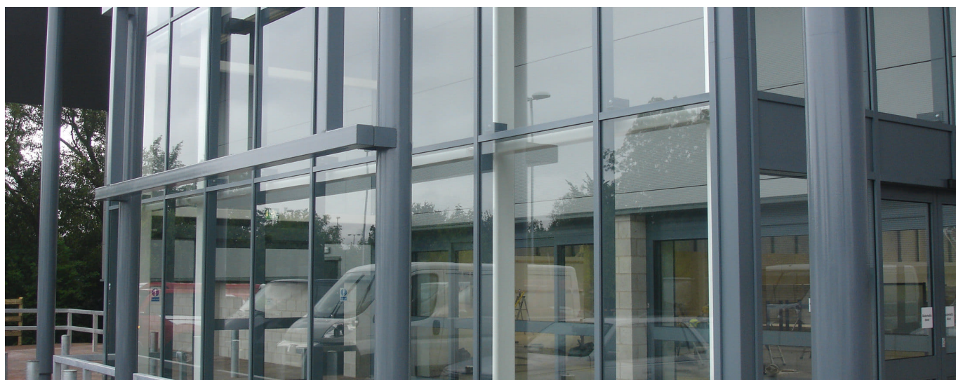
PROJECT PHOTOGRAPH A two storey grey aluminium curtain wall on a commercial building, with brick paving and bollards at the foot.
