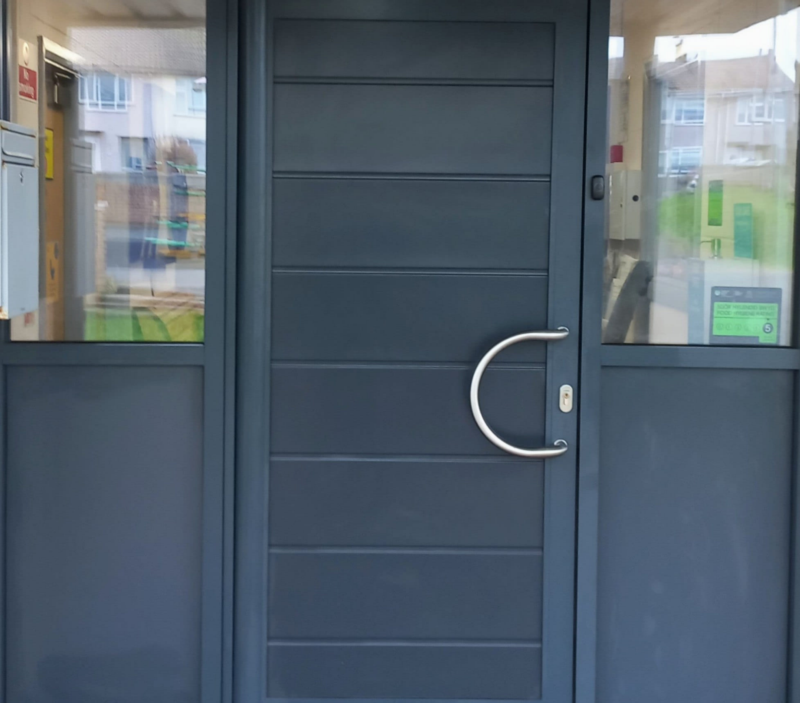
PROJECT PHOTOGRAPH An anthracite commercial entrance door with a bow handle, hung in a framed screen with glazed side panels.
