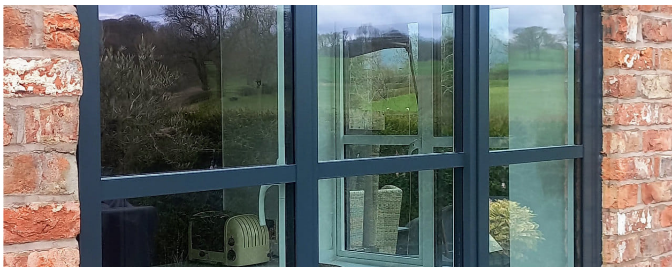
PROJECT PHOTOGRAPH A three light anthracite casement in reclaimed red brick, under a sandstone lintel and over a sandstone sill.
