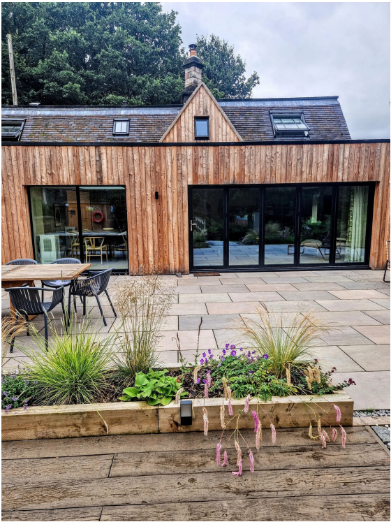
PROJECT PHOTOGRAPH Timber-clad extension, black aluminium bifolds, sandstone terrace.
