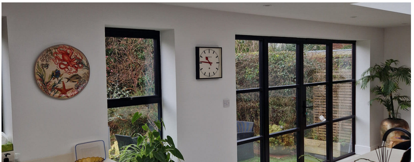
PROJECT PHOTOGRAPH A heritage screen and a tall narrow window with matching glazing bars, seen from a kitchen island under a flat roof lantern.
