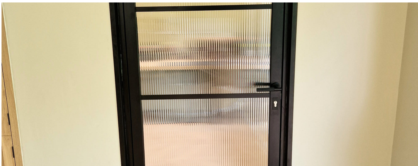
PROJECT PHOTOGRAPH A black steel look door with reeded glass and three glazing bars, hung against a plain wall.
